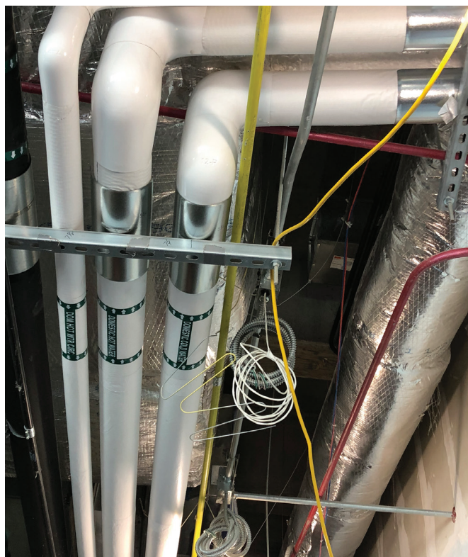
Insulation installed through clevis hangers
