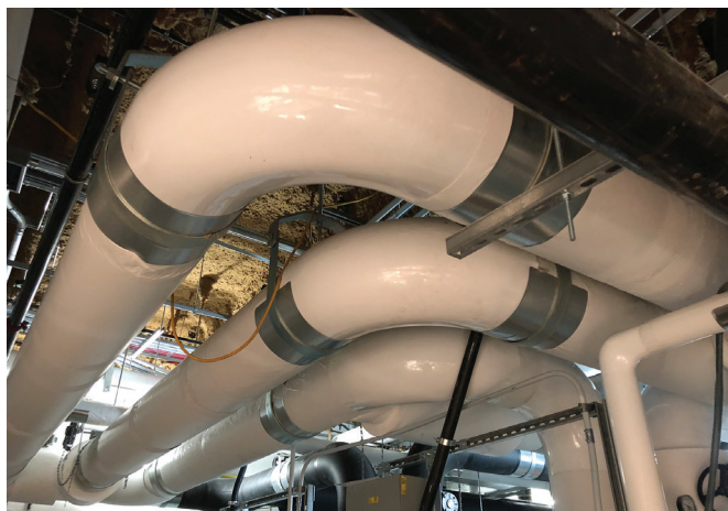
Ensuring adequate spacing for insulation between piping runs
